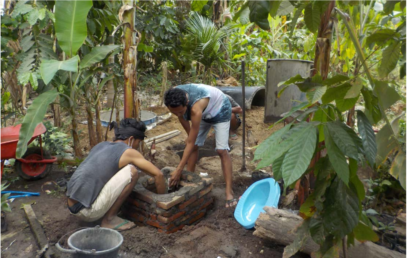
▲ Masons from PERSDAYGUN association are constructing closet for one of buyer in Lombok Utara district
