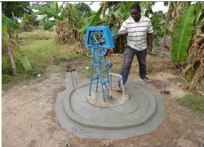
As training a tube well of 6 meters deep was drilled in 3 days and a Rope pump was installed.
