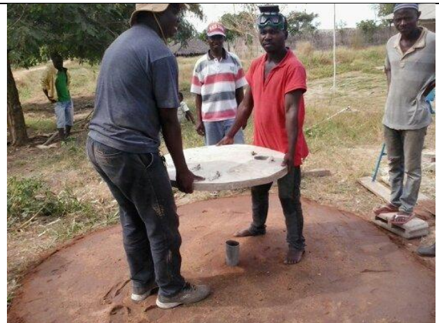
Installation of a well cover on a hand drilled tube well made during the training
