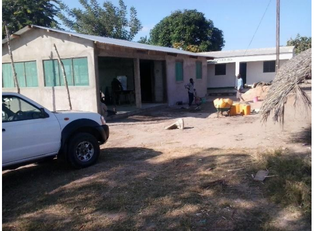
The Office and new trainings and production workshop in Bilibiza. This workshop is the only place with tools like a welding machine in the whole area.
