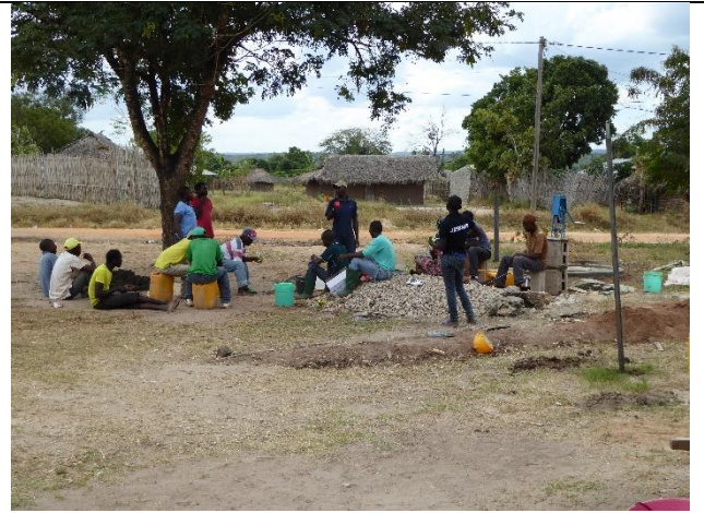
In front of the training centre a short tube well and a hand pump was installed.
