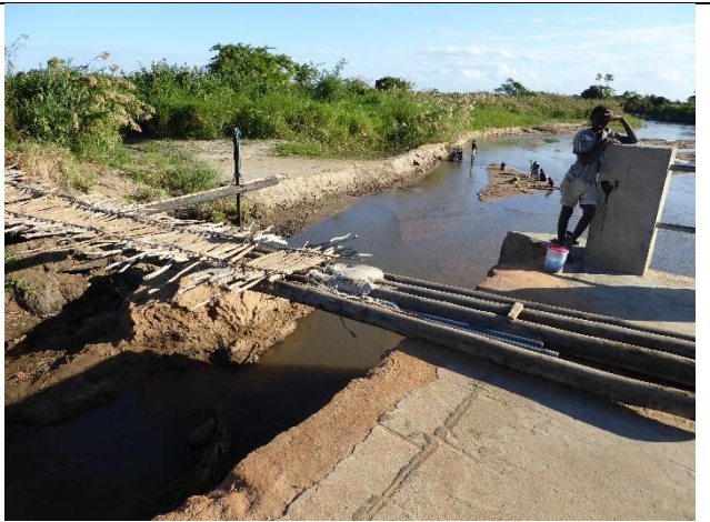
One of the bridges damaged by the floods
