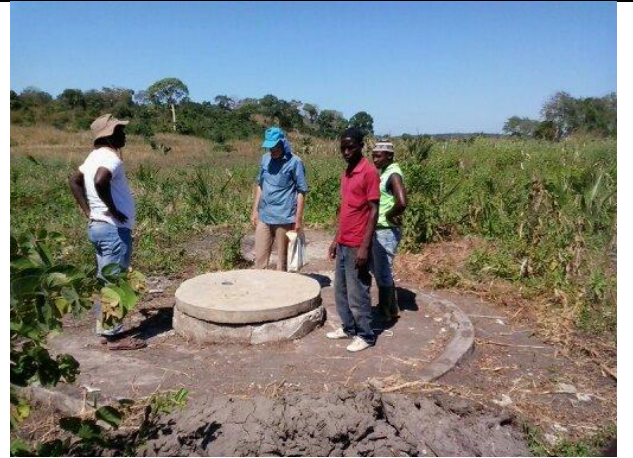
Near this water source there was a Rope pump installed which was washed away by the floods. Now an extra strong well and well cover is installed
