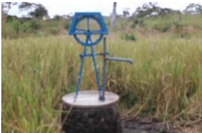
Figure 16: A drilled tube well and Rope pump installed for the vegetable garden
